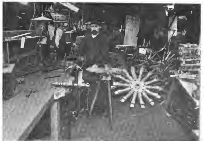
ASSEMBLING THE SPOKES IN THE HUB.
